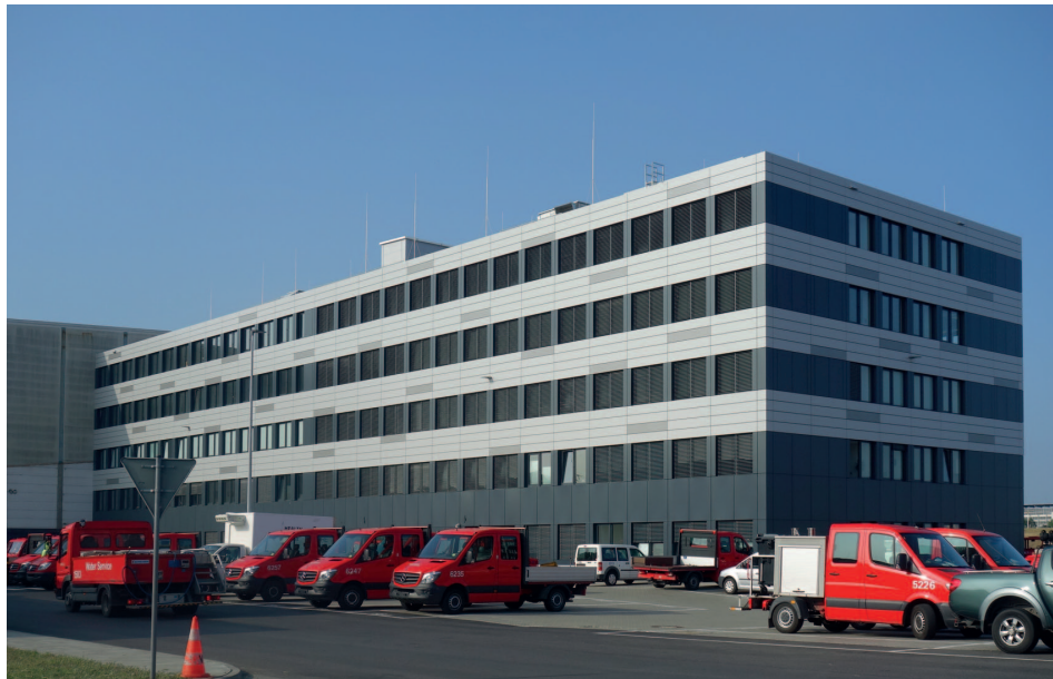
Fig. 6: The new ground handling building
